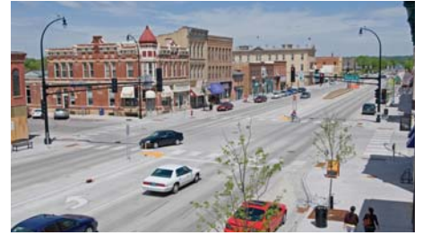
The project minimized impact to local drivers with a brief 133-day road closure.
