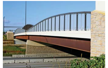
Well-planned construction ensured that traffic capacity was maintained throughout the process.
