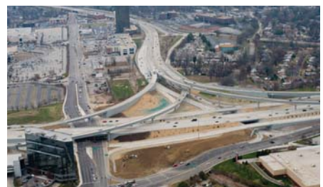
The project reopened to traffic nearly one month early and $11 million under budget.
