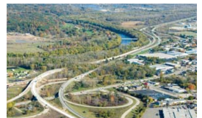
The on time completion of the project has relieved congestion for motorists.
